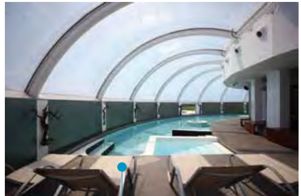
• ETFE cushions allow climate control inside the new zone.
