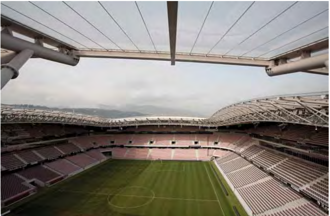
Innovative facade and inner ring constructed with ETFE sheets.
